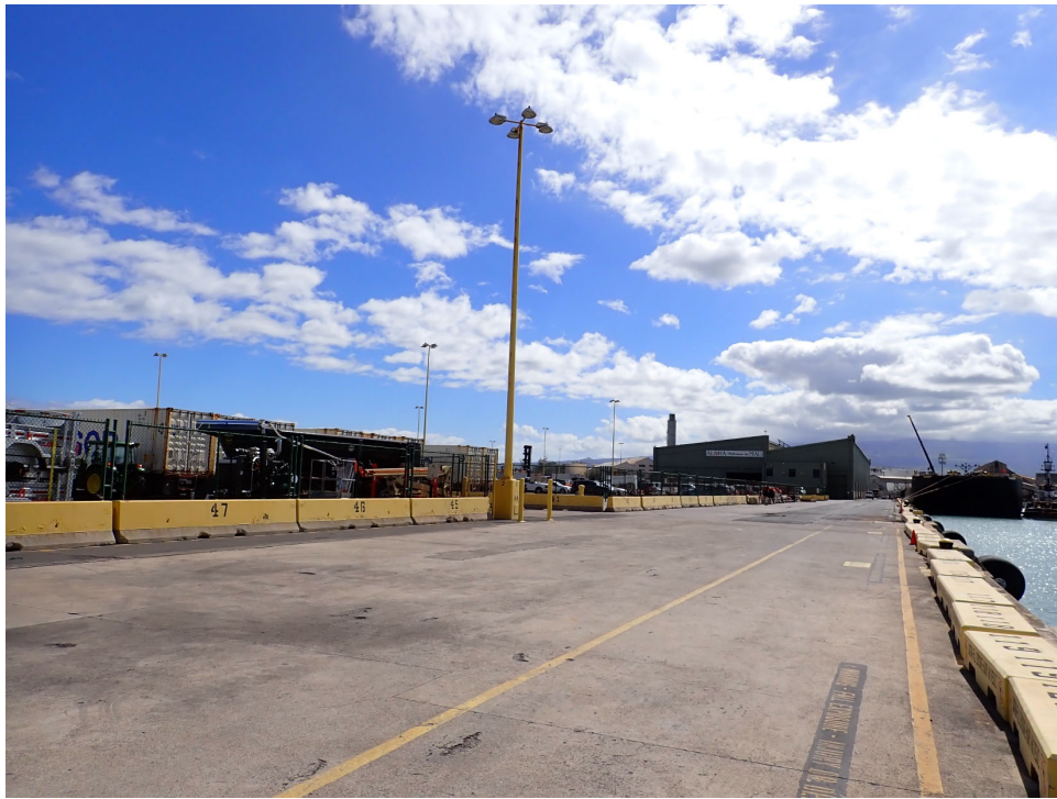
Photo 2: Project Site at Pole HM-2 at Pier 1. Pole has since been removed.
