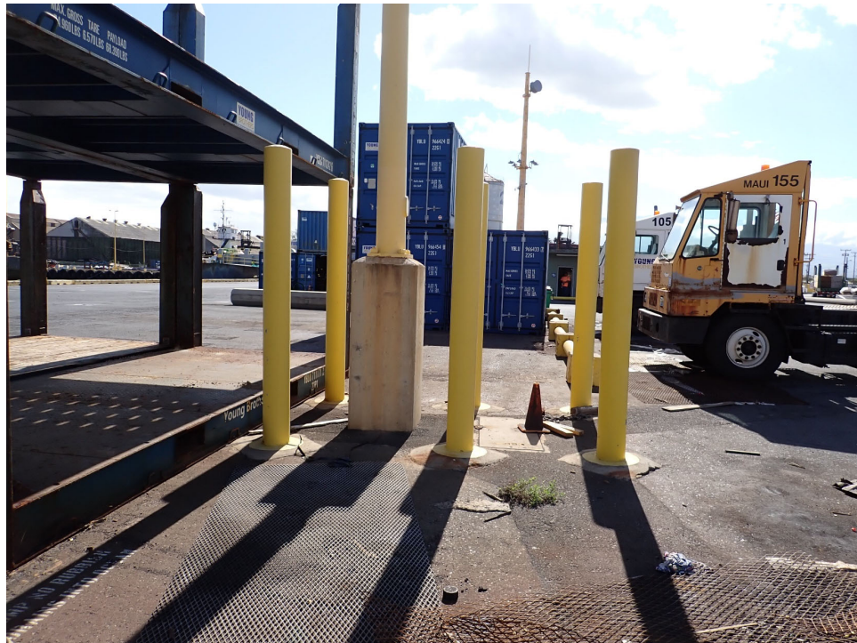
Photo 4: Pole SL-6 at Pier 2
