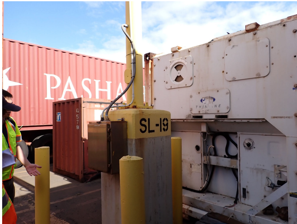
Photo 6: Pole SL-19 at Pier 2
