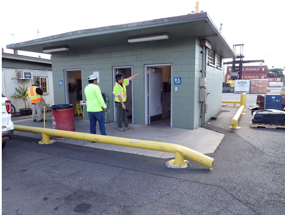
Photo 7: Comfort Station at Pier 2
